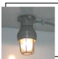
Explosion Proof Lighting
